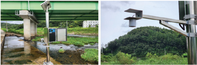
Flood prone road (Sejong City)
