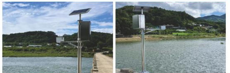
Flood prone road (Yeongwal)
